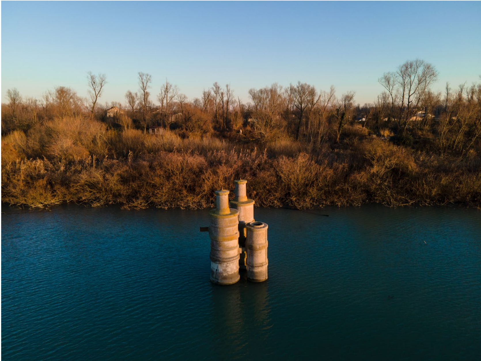
Ca' Pisani (Porto Viro, Rovigo). An old concrete well for extracting methane in the Po Delta. From the 30s, until the suspension of such activities decreed by the Government in 1961, billions of cubic meters of methane and natural gas were extracted in this area. The extraction took place from hundreds of wells (about 30 in the Delta) no deeper than 1000 meters. Through concrete infrastructure, the gas was sent to compression stations, while the salt water (1 cubic meter of water for each cubic meter of gas extracted) was discharged into the ditches and drains. The consequences of subsidence are easy to imagine: the lowering ground also dragged with it the embankments, which became thinner and less safe, adding to the water pressure on the levees and increasing the probability of leaks, overflows and even collapse.
