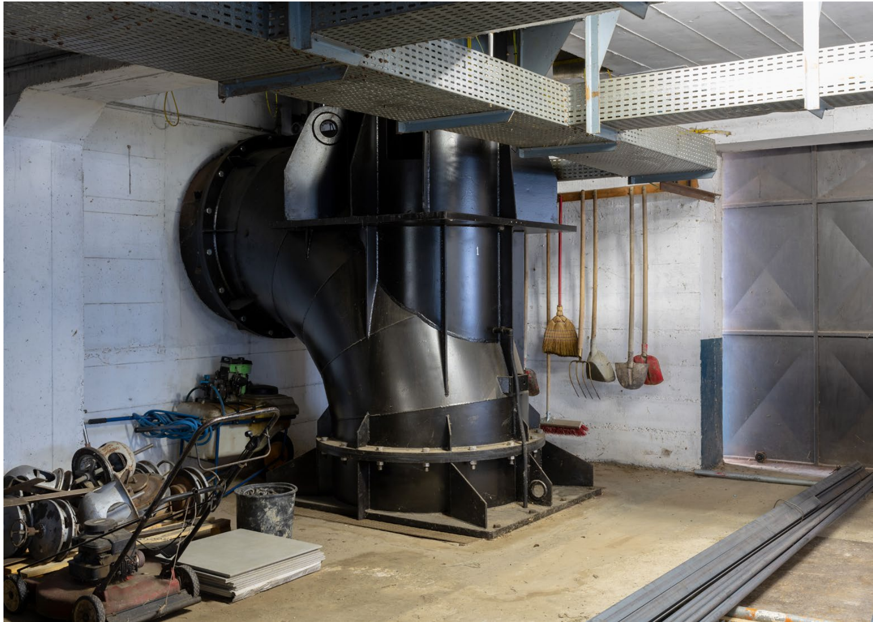
Gorino Veneto (Rovigo). Goro drainage pump collector. Built in 1977, it is one of the most recent and powerful systems, essential for ensuring the hydraulic safety of the entire Island of Ariano which channels water through the Veneto drainage ditch (Scolo Veneto). The plant became necessary at the end of the 1960s, after the natural compacting of the ground and the extraction of methane lowered the level of the watercourse that once flowed into the sea, next to the Po in Goro, through an outflow bridge with sluice gates.
