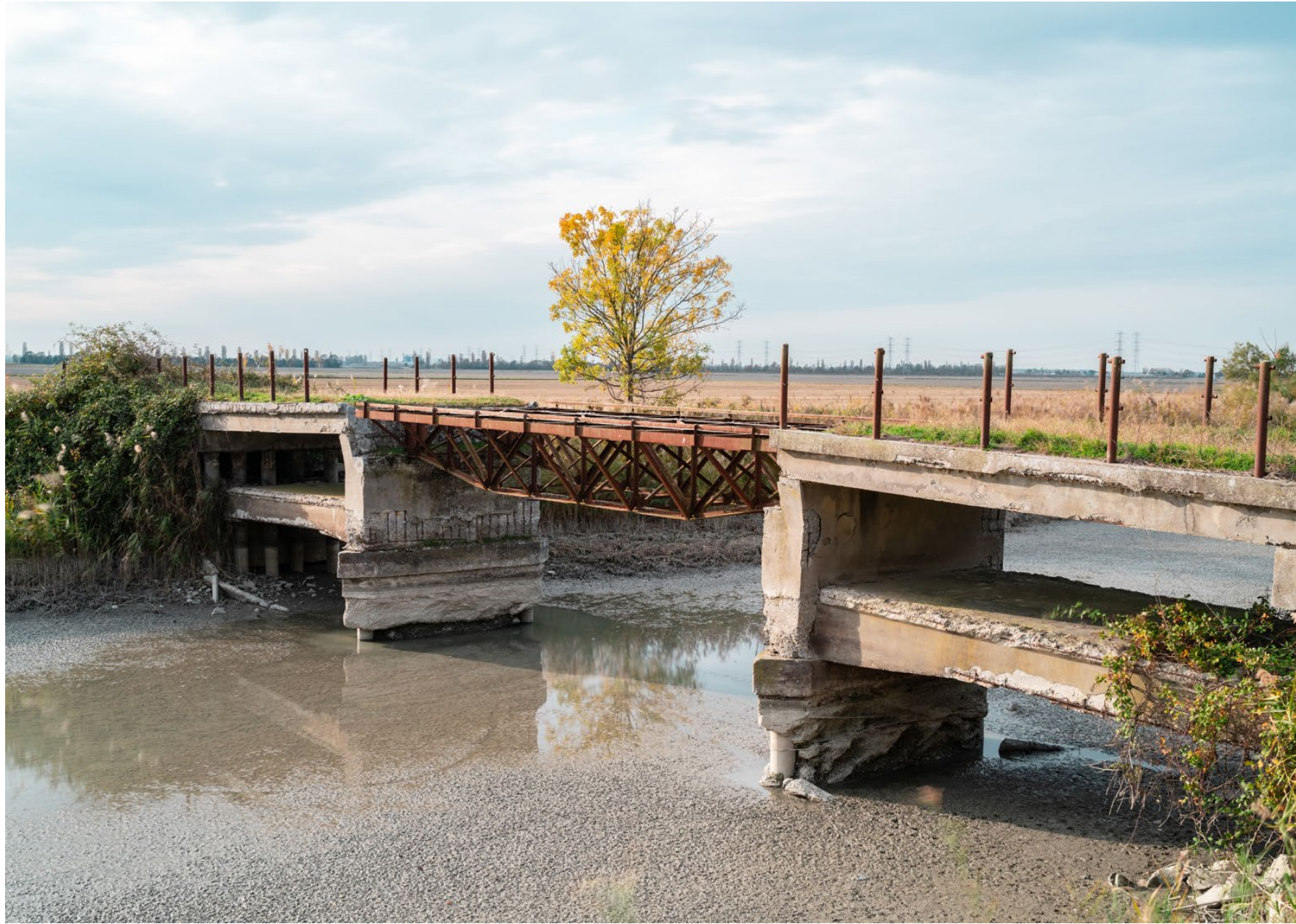
Ca' Mello (Porto Tolle, Rovigo). The famous “Ponte Colpi” which has a very peculiar architecture. A second bridge was built on top of a previous one that decades earlier had sunk below the water level. The bridge is one of the many works that have been required over the years to adapt structures and embankments to cope with the progressive subsidence of the ground.
