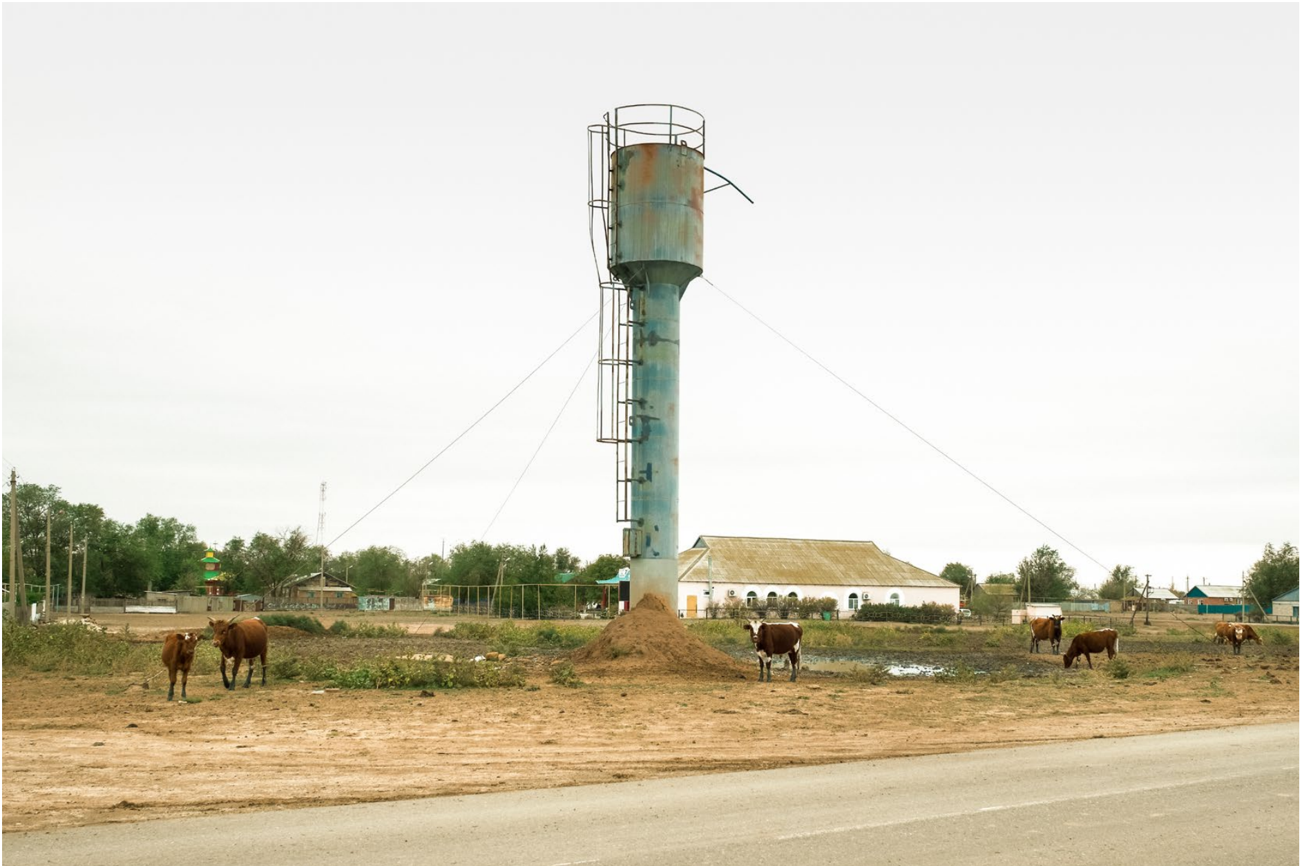
A huge water tank in Adyk, 150 km from Élista. The tank is connected to a purification plant that makes the ground water drinkable, thus counteracting the dramatic shortage of water resources afflicting the local community.
