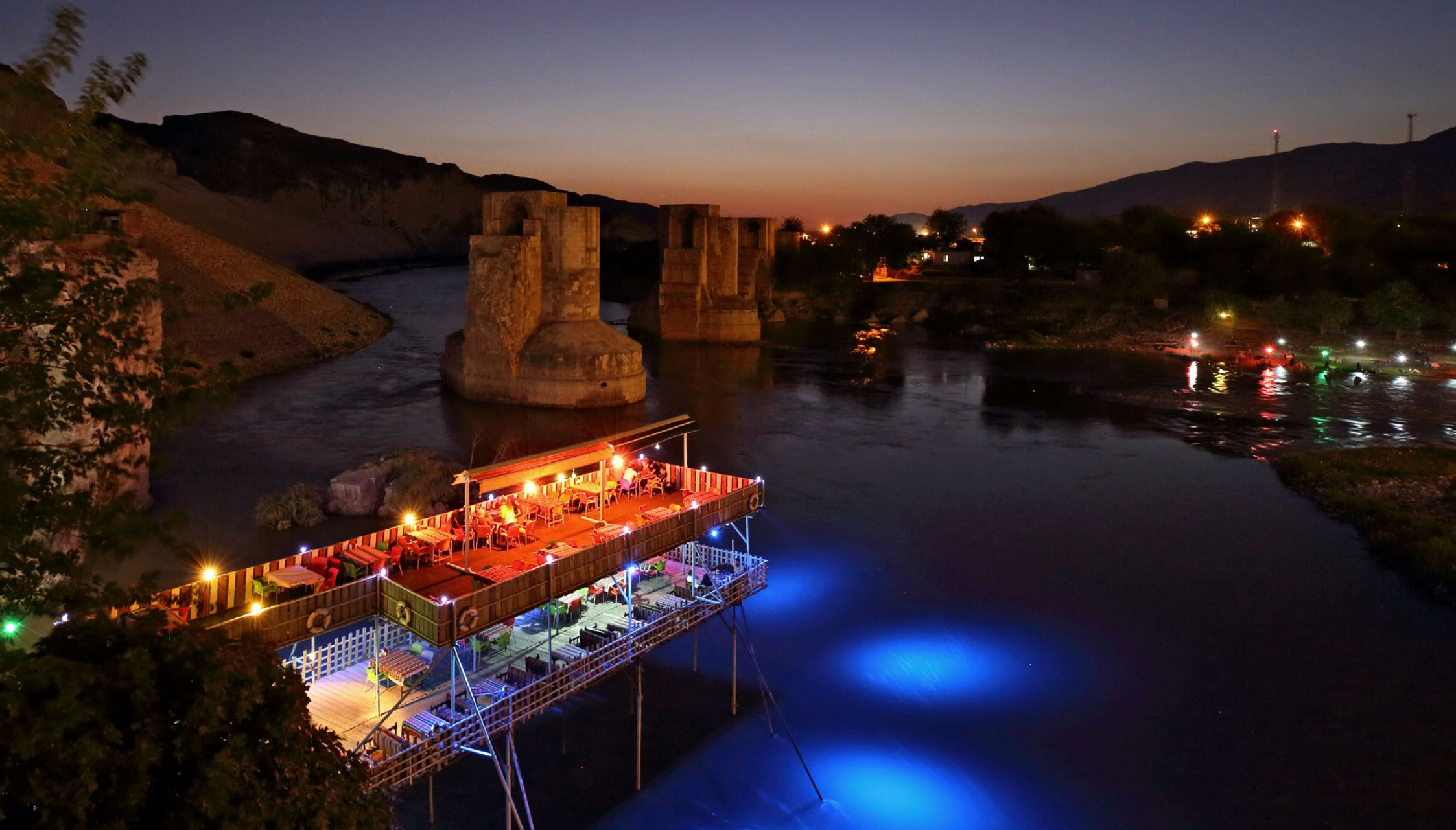
Twilight over the Tigris with the pylons of the 12th-century bridge and the premises of the old Hasankeyf, which were flooded after the activation of the Ilisu dam. (2019)
