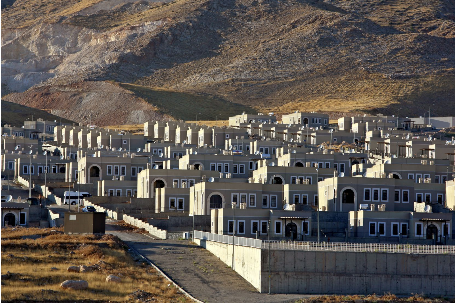
A panoramic view of buildings in new Hasankeyf. (2019)
