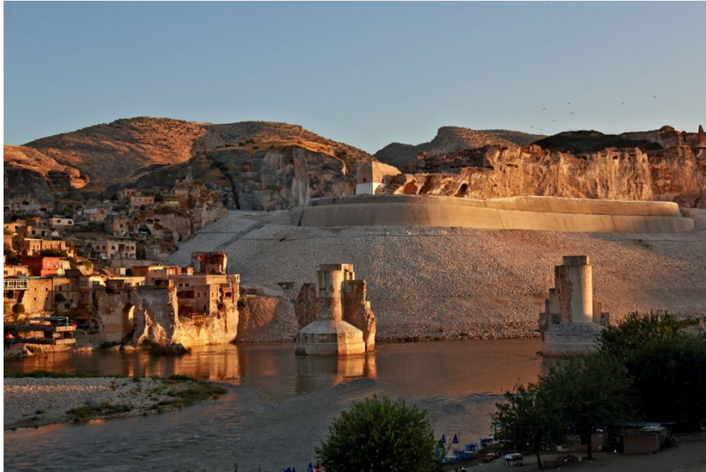
A panoramic view of Hasankeyf, the pylons of the bridge over the Tigris built in the 12th century and the wall built to protect the cliff from the arrival of the waters of the lake. (2019)
