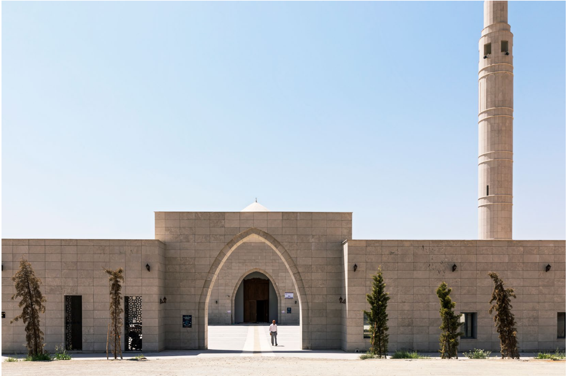
The new mosque built in the modern settlement of New Hasankeyf. Some of the families whose homes were submerged beneath the waters of the reservoir, created as a result of the controversial Ilisu dam on the River Tigris, have been relocated to the new settlement. Part of the archeological area has also been submerged. (2021)
