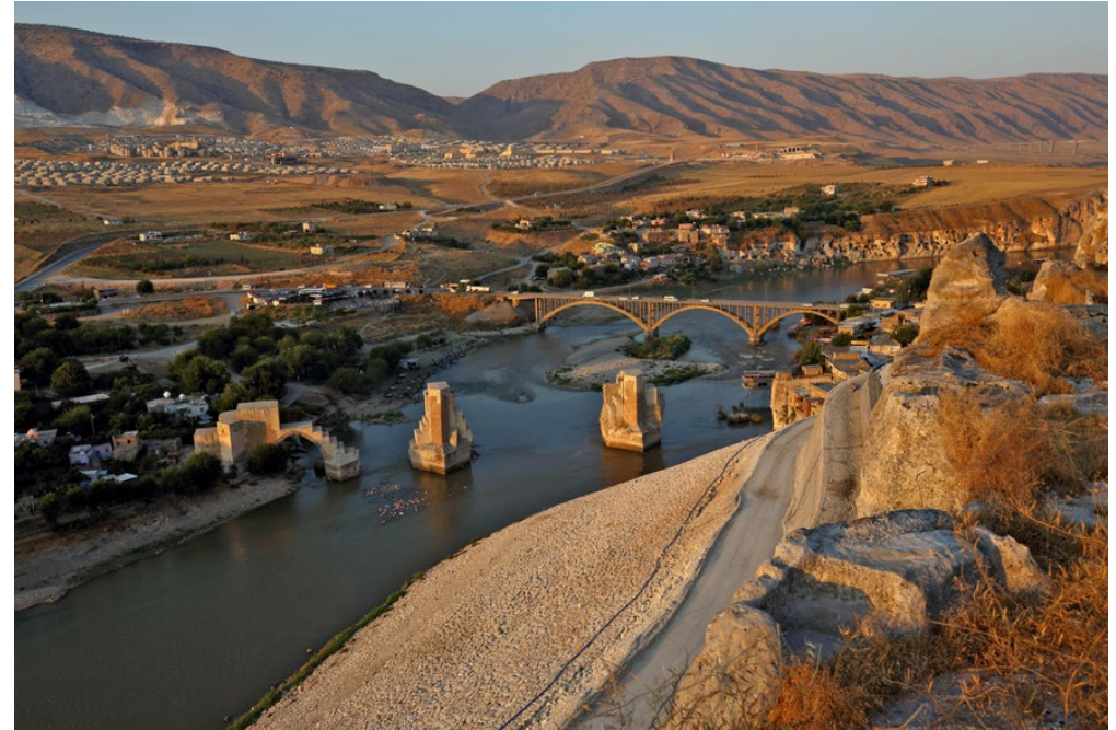
Hasankeyf, the pylons of the bridge over the Tigris built in the 12th century and the wall built to protect the cliff from the arrival of the waters of the lake. (2019)
