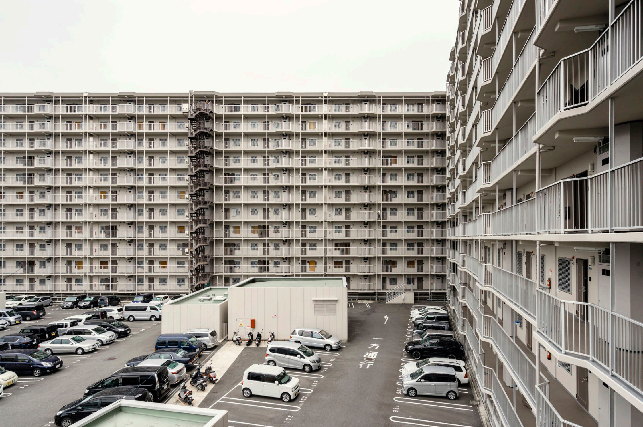
Osaka, Ikuno-ku ward, a large residential complex, at its centre is a resident's parking area.
