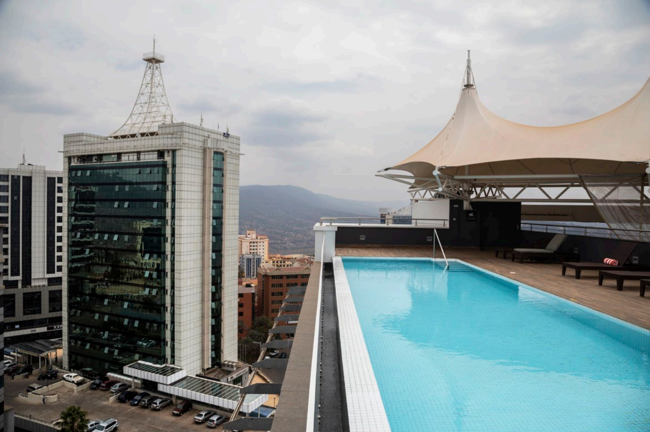
A rooftop swimming pool in one of Kigali's luxury hotels.
