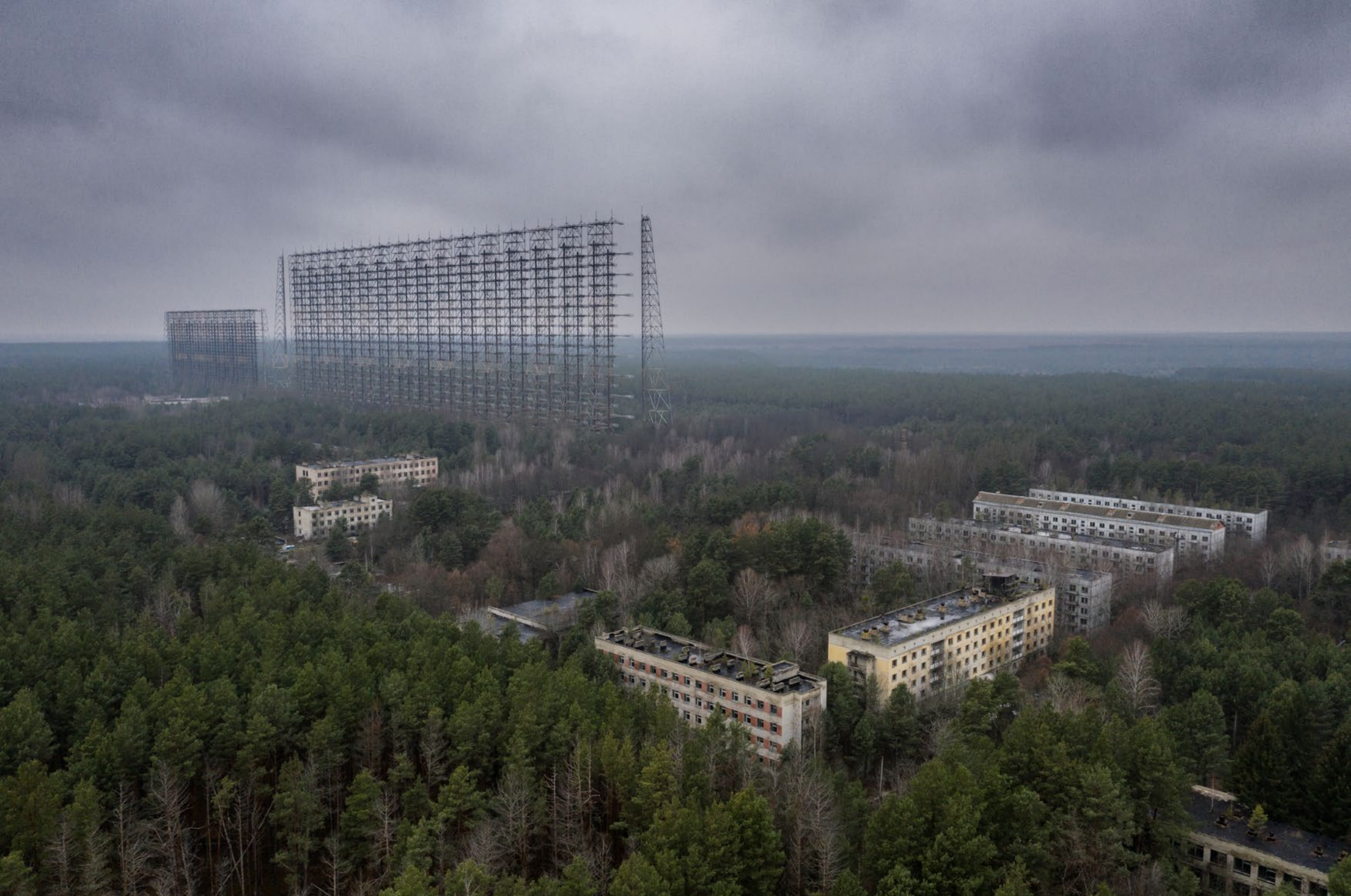
Chernobyl Exclusion Zone. The Duga 3 military antenna is a huge radar antenna 150 meters high and 500 meters in length with buildings, and was part of the anti-missile defence system that would track any missiles from the USA.
