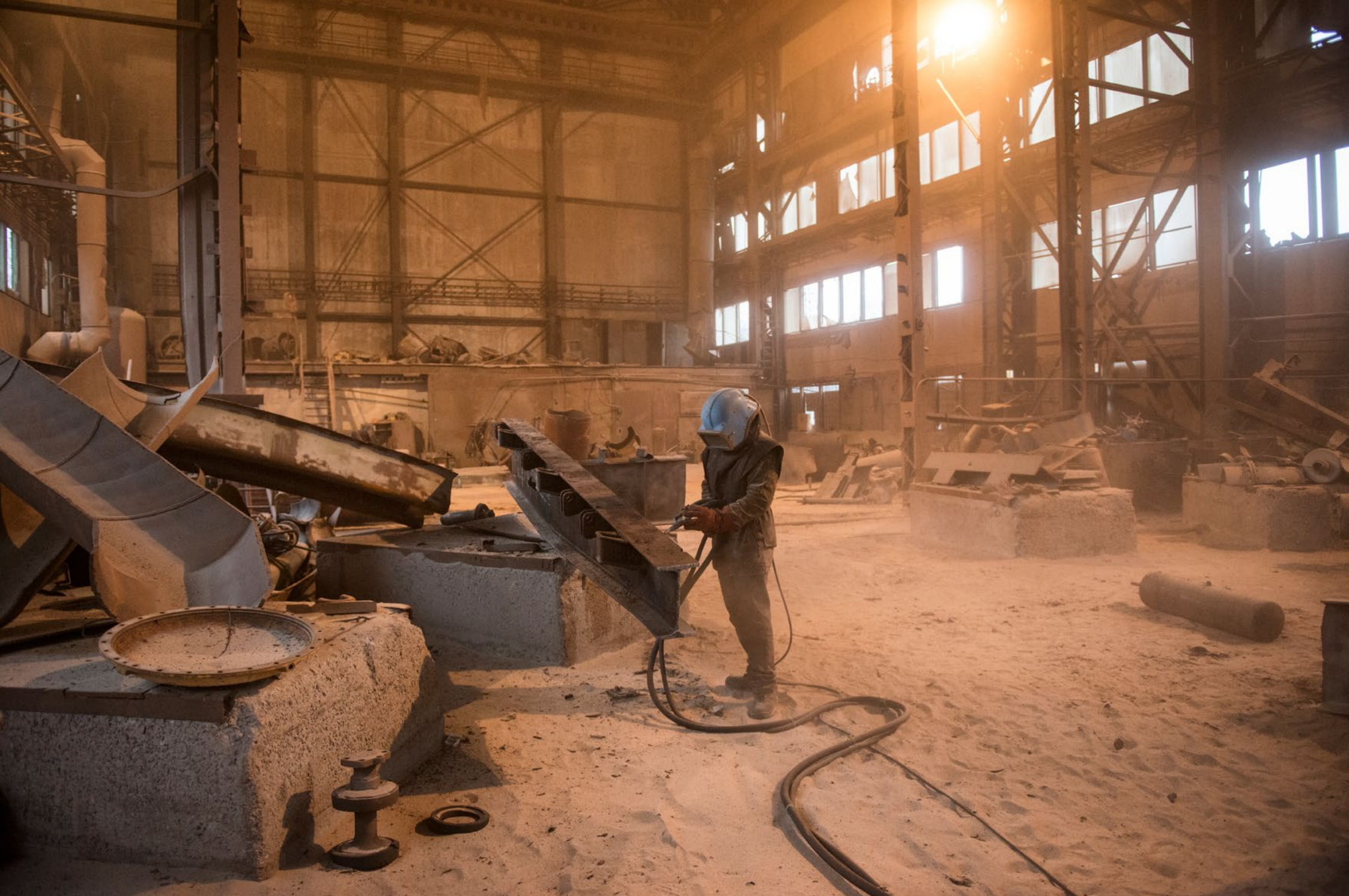
The hangar close to Reactors No. 5 and 6 where the scrap metals are cleaned of radioactive particles and recycled. There is still a million of tons of rusty metal abandoned in the Exclusion Zone. Recycling all this metal is a billion US dollars business. Workers operate with minimal protection, even though it is mandatory, moving around for hours in the middle of toxic clouds. Their work is terribly dangerous, almost a death sentence in slow motion.
