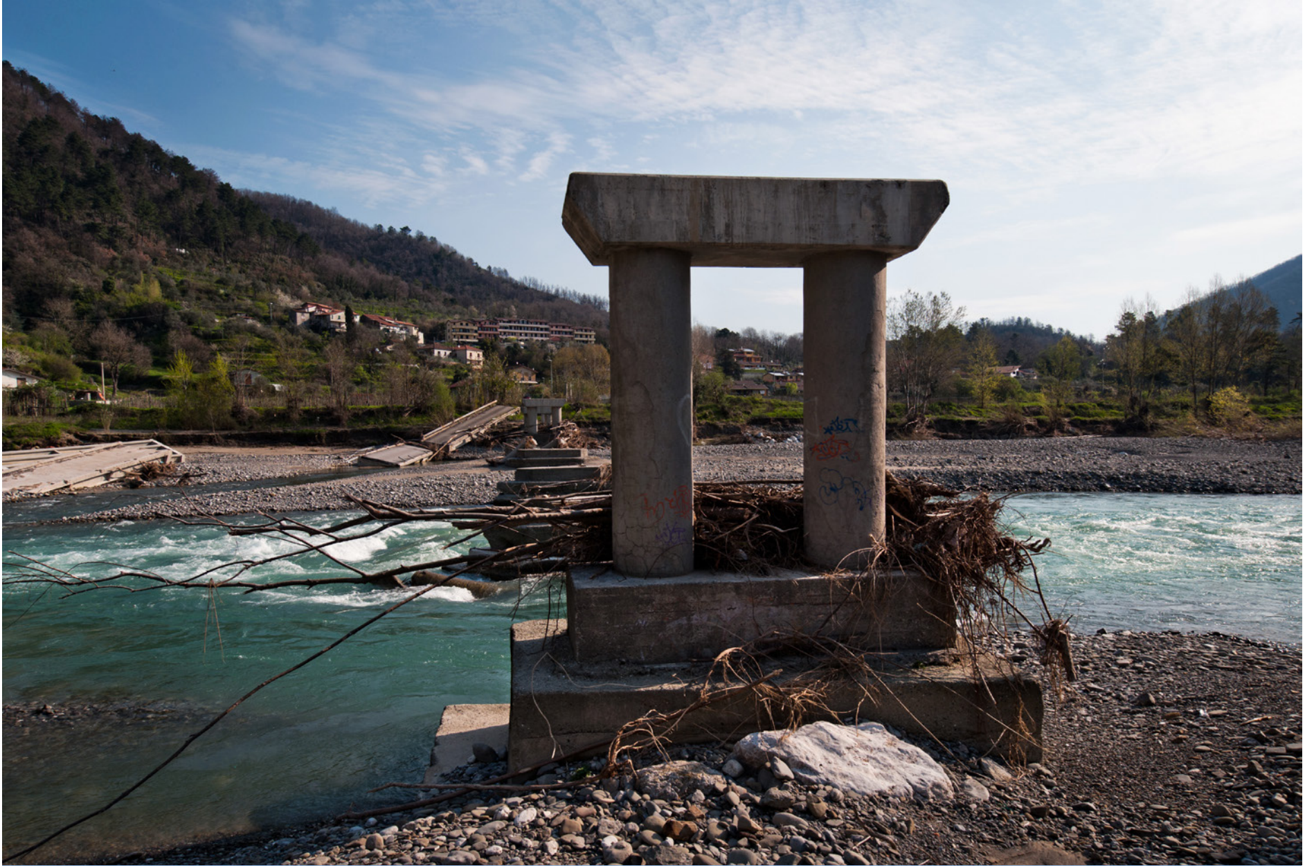
Aulla (Massa Carrara, Italy), this bridge, which broke into pieces after a flood, used to connect Stadano with the road to Aulla. In recent years water bombs and cloudbursts have increased considerably in Italy, causing damage to agriculture and confirming the inexorable tropicalization of the climate.
