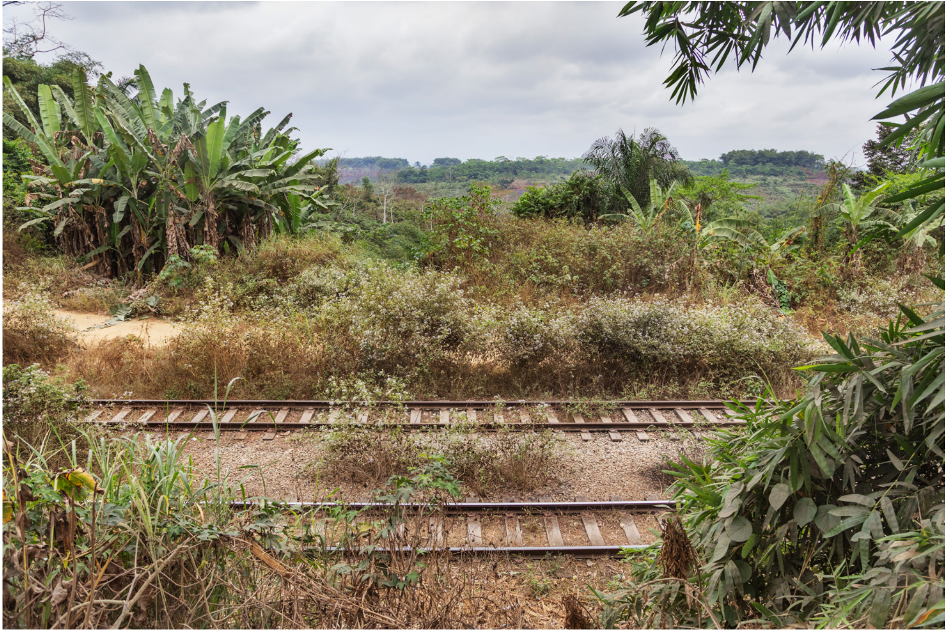
Pointe-Noire (the Republic of Congo), rail tracks at Hinda. The section of railroad connecting Pointe-Noire to Brazzaville was built in the early 1900s and was a symbol of development and prosperity. Later it was virtually abandoned and is now used sporadically for freight transit.
