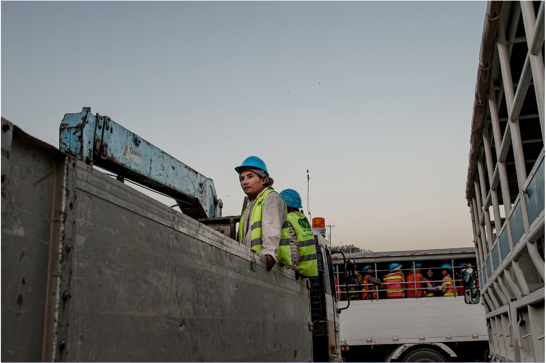
Xayaburi dam (Laos). Worker on the dam construction site. Laos plans to build around 140 dams on the Mekong and its tributaries in the coming years, half of which will be financed by China, with the ambition of becoming "the battery of Asia" (2013).
