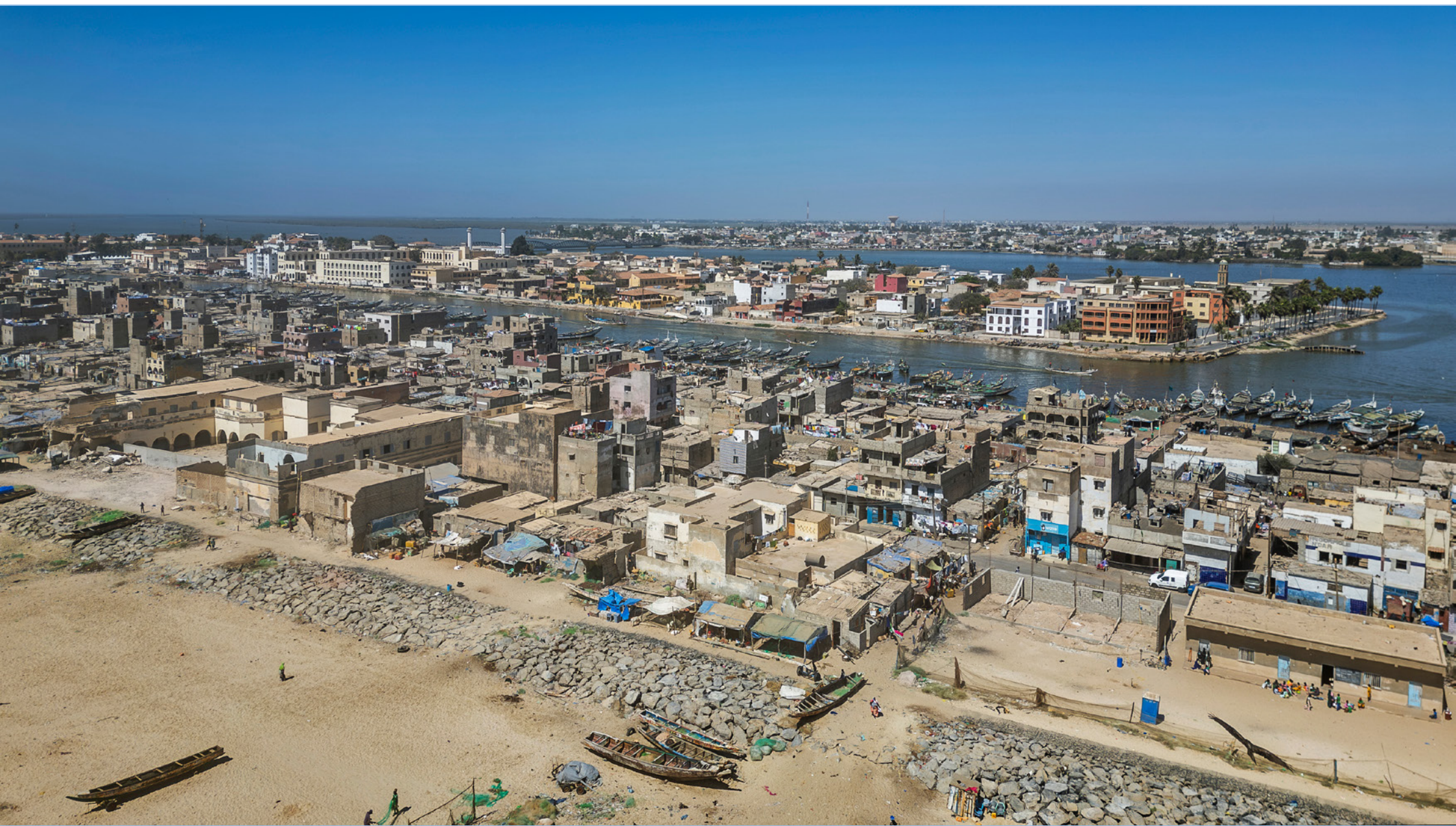
Senegal, St. Louis – Overview of the fishing district of Guett Ndar. In the foreground, the embankment built to protect the houses from the rising sea waters, in the background, the historic core of the city founded by the French on an island in the river.
